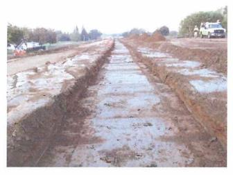
During this time period Magnus has worked on the removal of spoils associated with the cutoff wall production from the site and exposing the top of the cutoff wall along the elevation 40' working platform so that embankment can commence at that location.
